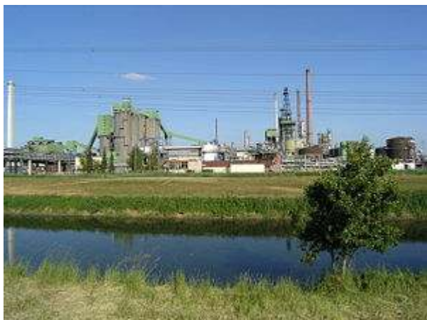
MiRO refinery at Karlsruhe
